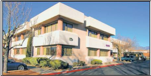
COURTESY OF ARGUS INVESTMENT REALTY BGK Group has dropped its asking lease rate at Seagull Office Plaza, shown here at 5801 Osuna NE, by 22 percent.
