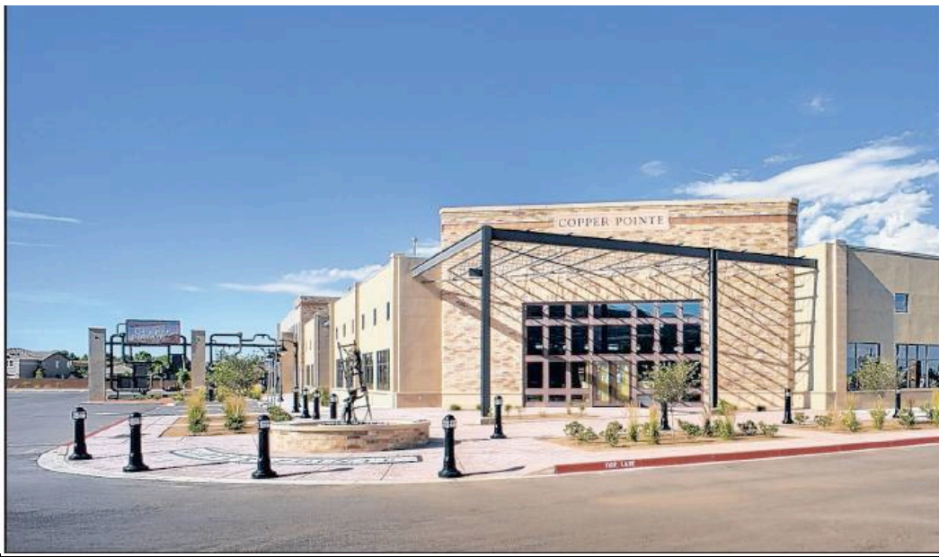
COURTESY DEKKER PERICH SABATINI COPPER POINTE Copper Pointe, the 211,077-square-foot overhaul of the former Siemens Stromberg-Carlson plant near Interstate 40 and Eubank NE, attracted a private college as its first tenant in late 2009.
