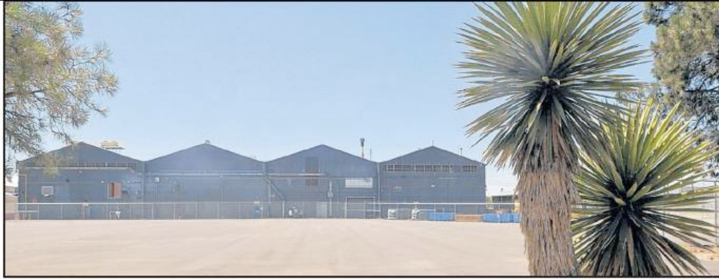
JOURNAL FILE As a sign of the times in the industrial market, General Electric's 477,000-square-foot aircraft parts plant in the South Valley is scheduled to close later this year.
